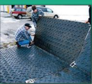
Steel links lock mats together to form a semi-permanent, yet portable, continuous roadway, walkway or working platform.
